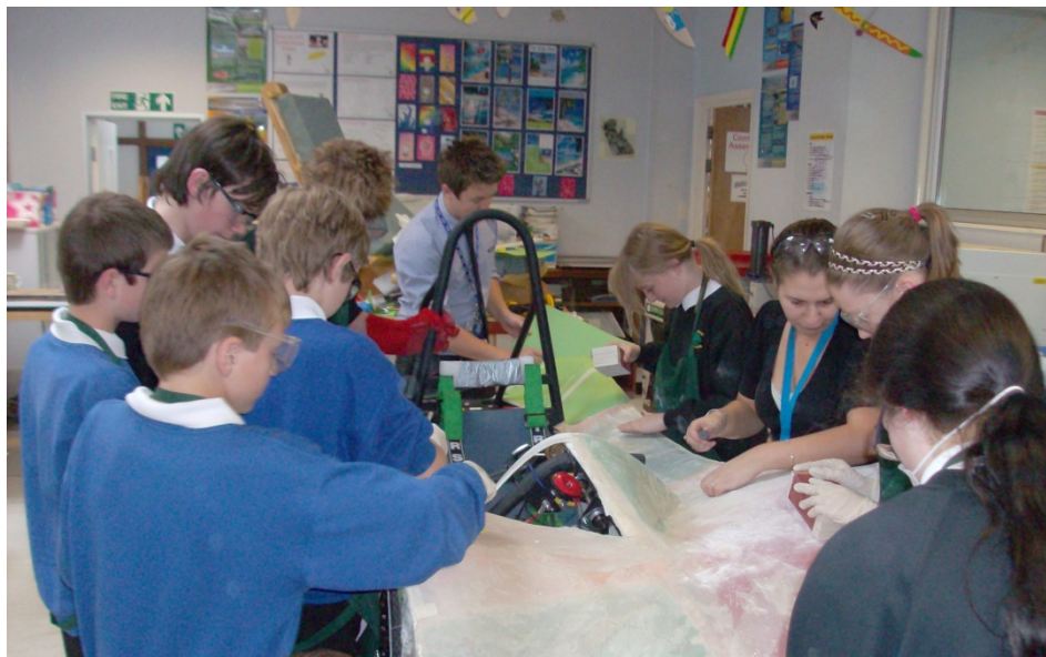
We then painted the bed sheets with a fibreglass resin which hardened the bed sheets, creating our bodywork.
